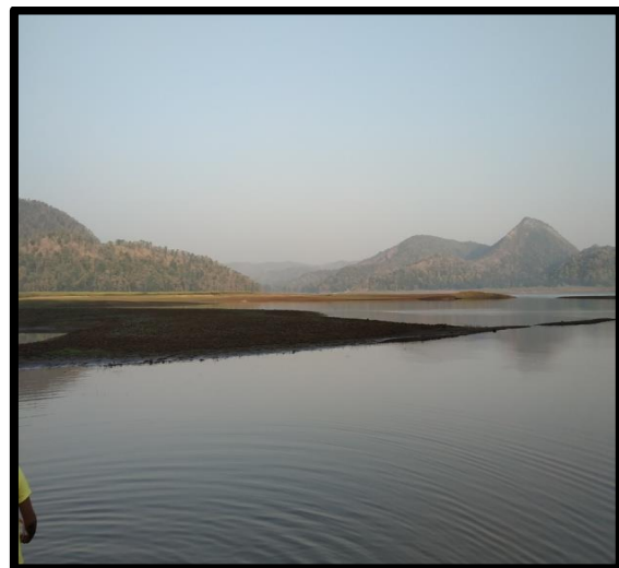
Plate.2. View of Station-II (back site of Dam)
